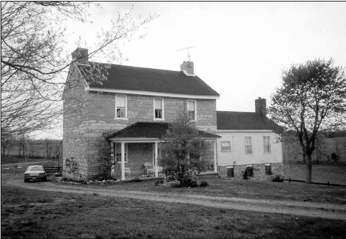
Figure 4. View of the Thompson House. [Note: This house is constructed with much larger pieces of stone than the Miller house or McConnell's Homestead but the layout and general appearance are similar. The walkout cellar door of the Thompson house is not visible in this picture because it is located on the right gable end toward the backside of the house. There also were cellar windows that are now below grade.]
