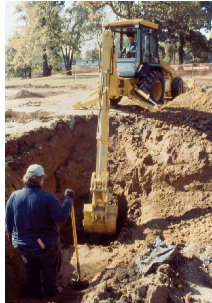
Figure 5.59. Phase III backhoe excavation of Feature 10, the well, looking west
